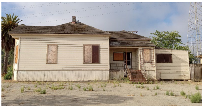
Snyder Hammond House (front entrance, north side)
